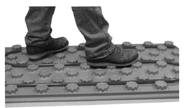
• Other than ensuring the PEX is securely in the panel when making a corner, installation is as simple as walking the tube into place.
