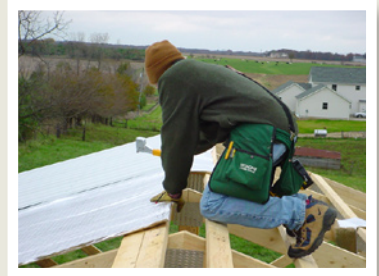
Installs with staple gun
